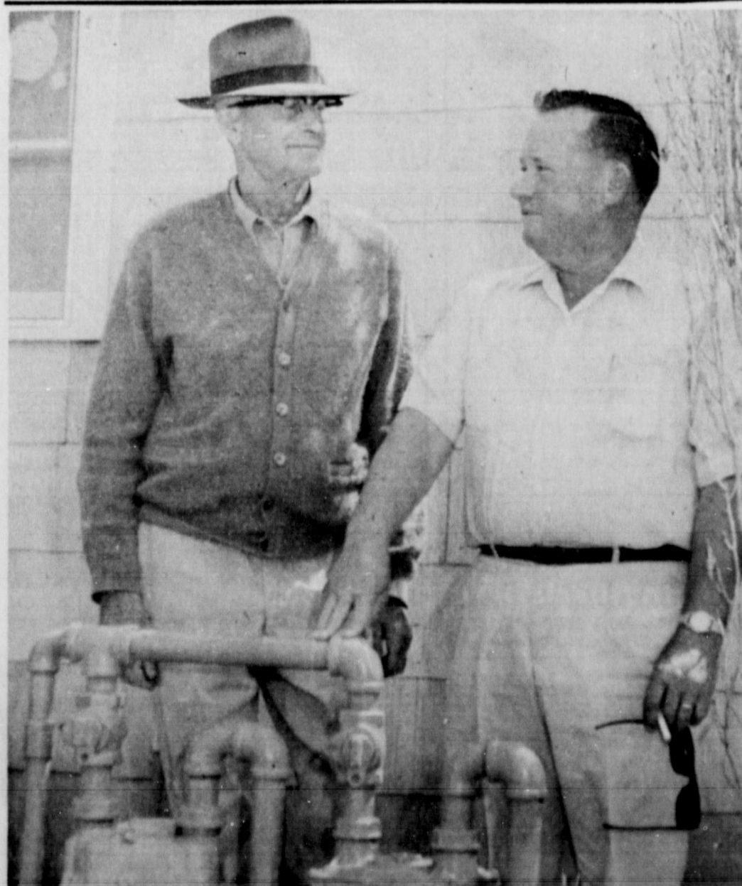
1,000th METER . . . Ralph Shirley, right, and A.H. Hadley, are shown beside a meter installed recently by Pioneer Natural Gas Company, which was the 1,000th gas meter within the City of Friona. The meter was installed at Hadley's duplex.
