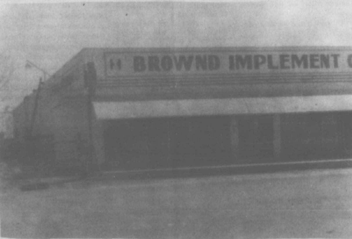
G & C Auto is moving to a larger building. Shown above are roofers putting on new roof on the building where Brown Implement was once located.
