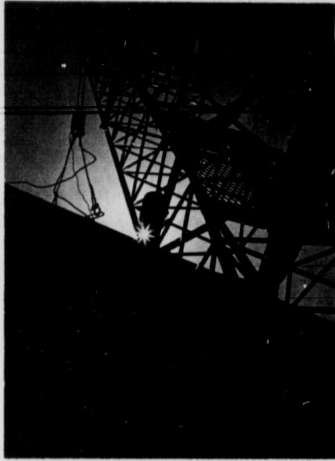
EQUIPMENT INSTALLED . . . Pictures above show the installation on Monday of a 70-ton feed bin at Hi-Plains Feed
