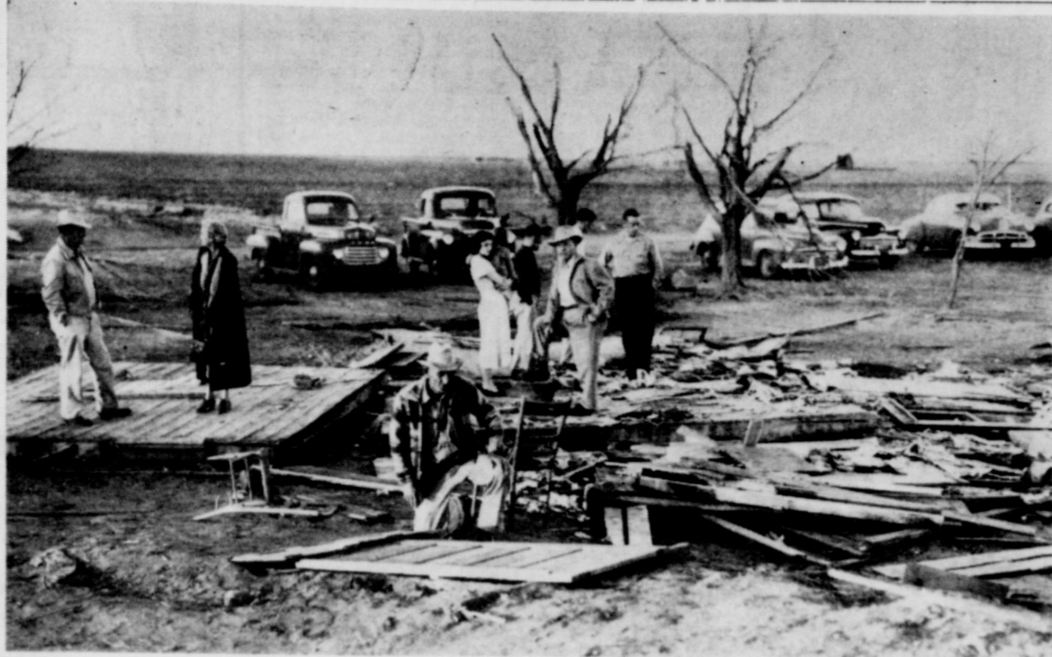
TORNADO SMASHES HOME NEAR WHITEFACE —The unbelievable damage left by a tornado which struck the Fairview community early Saturday night is visible in the photo above. The picture shows all that was left of the Raymond Reed home seven miles north of Sundown. Eight persons were huddled on the floor, at left, when the storm had passed. Mr. and Mrs. Reed, their three children, Reed's brother, Jack, and his wife, and a Mr. and Mrs. Kester, mother and step-father of the Reeds. Kester
