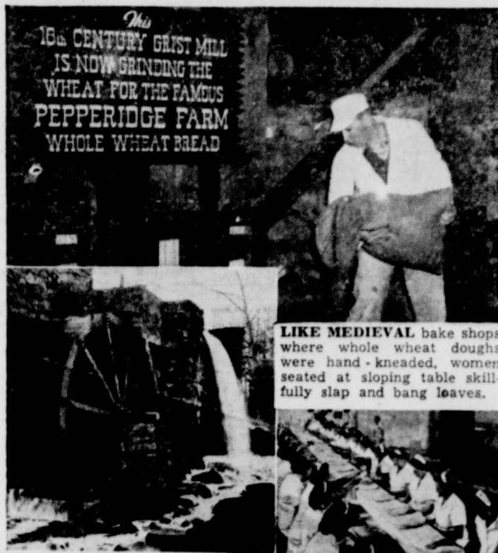
OLD WHEEL that turns by water power is characteristic of mill where burrstones turn slowly and crush grain. Flour retains the live wheat germ.
