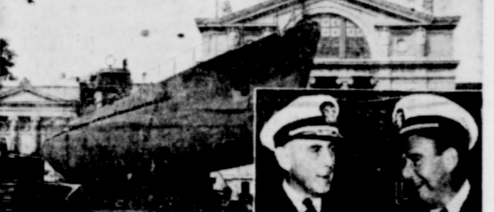
Jacked up four and one-half feet above beach pier, sub was then rolled across Outer Drive to permanent exhibition site at the east wing of Chicago's Museum of Science and Industry. Actual capture of sub took less than 20 minutes. Moving it to final berth, a distance of 547 feet, took 40 days. (Inset) Present for dedication ceremonies were Rear Admiral Gallery and Commander Arthur Godfrey USNR.
