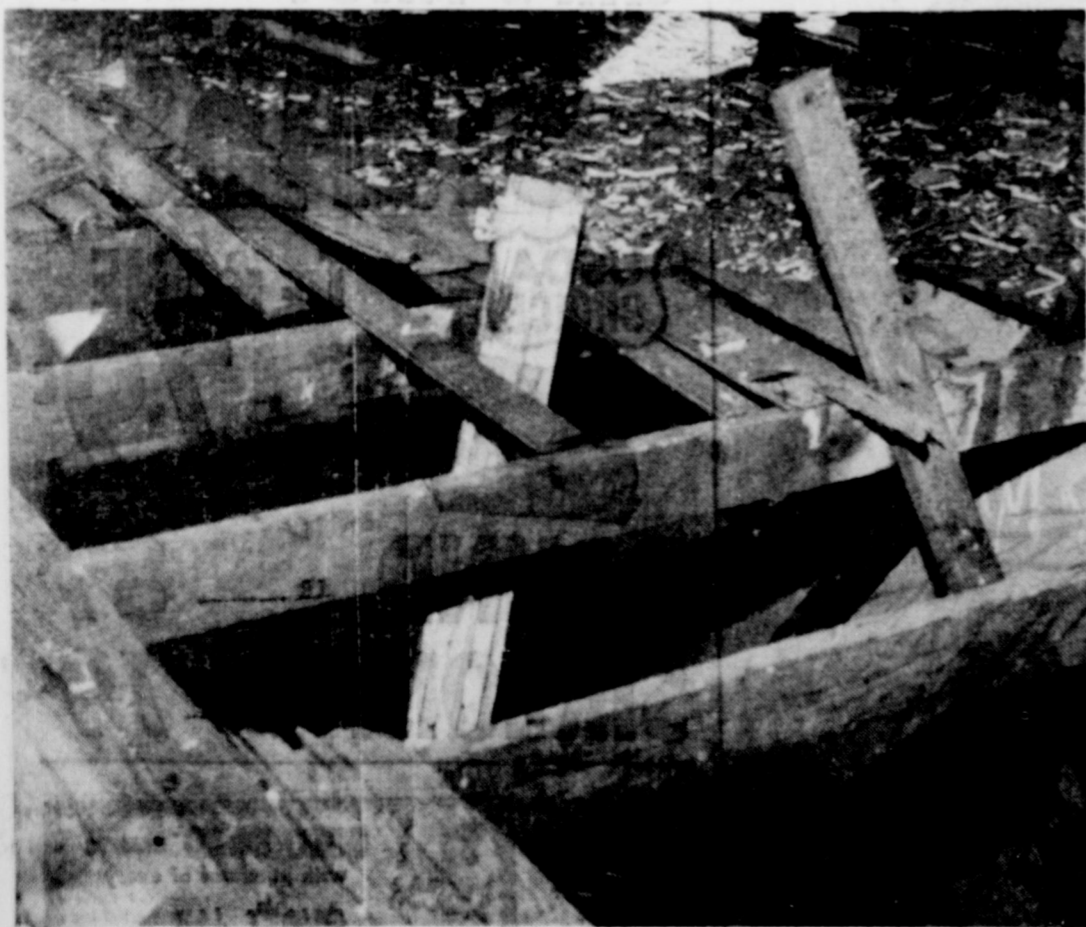
A child trap . . . BROKEN FLOORING in an abandoned house reveals a gaping hole that could easily result
