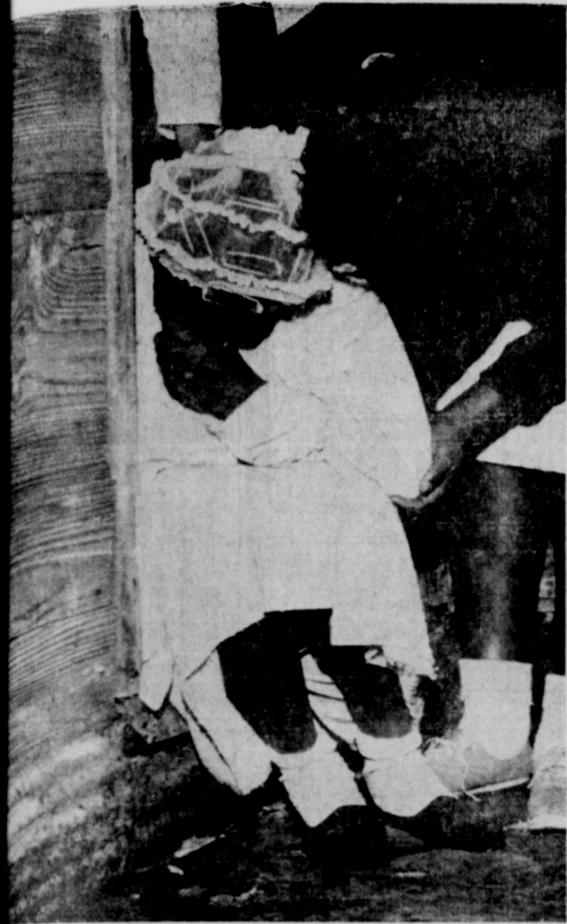
solation after the fire . . .
