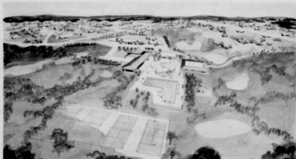
The Highland Lakes Recreation Center, being built at a cost of almost three quarters of a million dollars, is the center of outdoor recreation and family fun. Its country club facilities include an 18-hole championship golf course and an Olympic size swimming pool.
