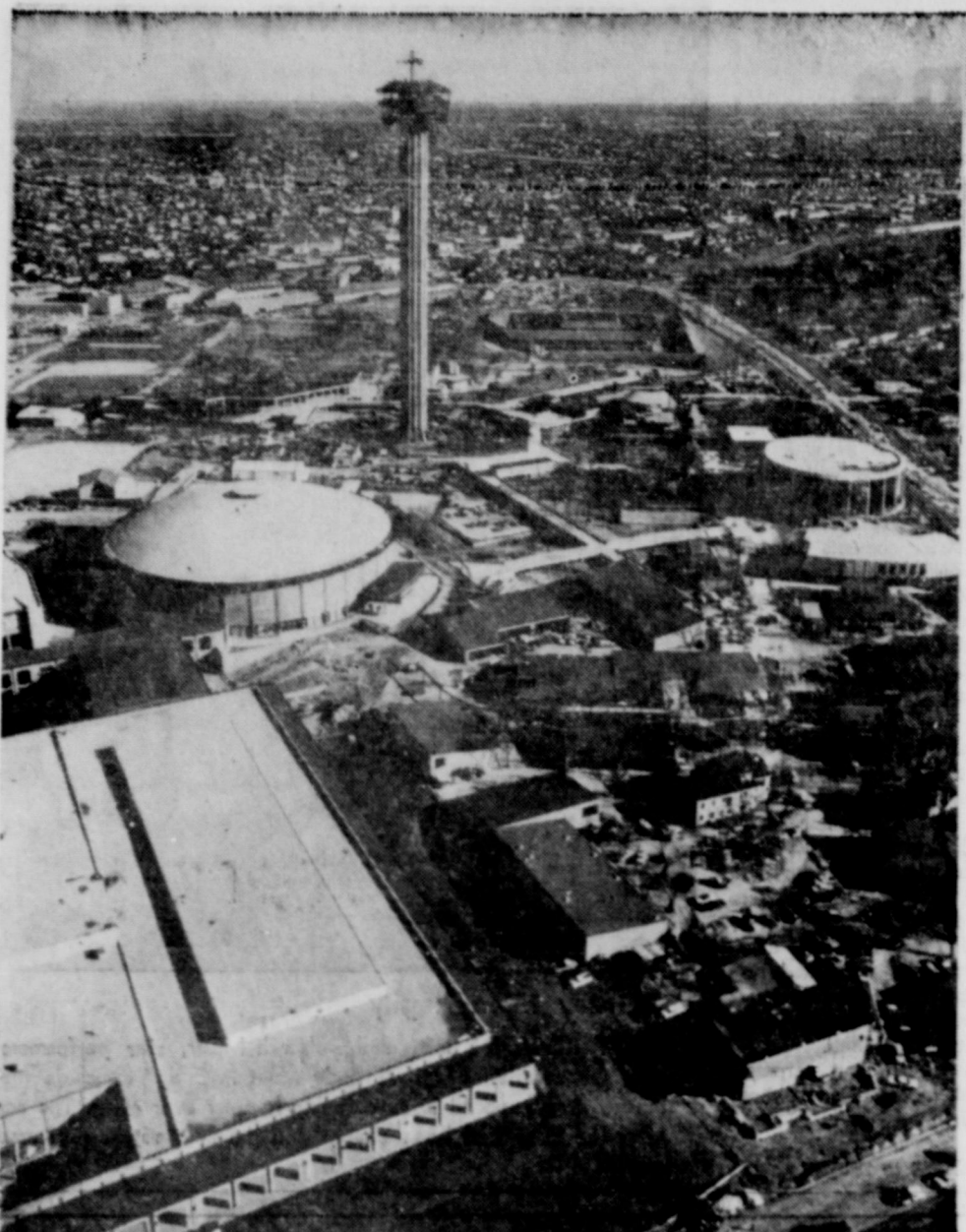
WORLD'S FAIR—HemisFair '68, only a dream a few short years ago, stands proudly in San Antonio as the last month of work continues before the April 6 opening. The $13 million civic center complex in the foreground, 622-foot Tower of the Americas in the center and the $6.75 million United States Pavilion on the right center are all prominent in the picture of the 92.6-acre showcase.
