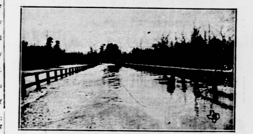
This photo shows water going over Highway 35 between Lufkin and Nacogdoches, Texas, for the first time since construction of the road 11 years ago. Traffic on this main highway between Houston and Shreveport was held up for some time when the Angelina River rose to unprecedented height.
