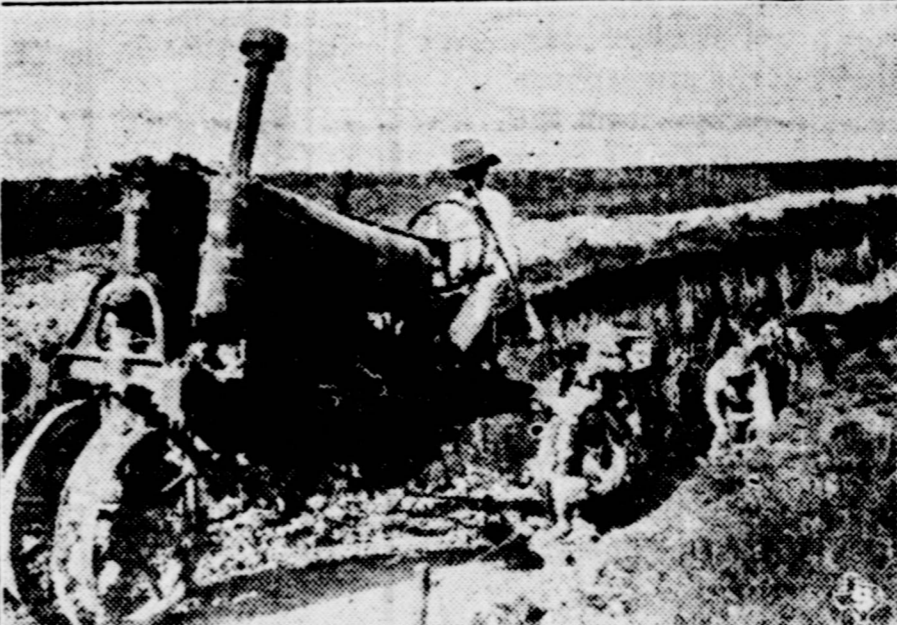
Here is A. D. Kaiser, DeWitt county farmer, who is shown digging a trench silo on his farm in Lone Tree community. Kaiser has found this method cheapest in storing his red top cane. The silo, when completed, will be 10 feet wide, 10 feet deep, 110 feet long, and will hold 80 tons of cane. The walls will be plastered and the top will be dirt in crown form to shed water. Seventeen of these silos are being built in DeWitt county this year, after two proved successful last year, according to J. A. Oswald, county agent.
