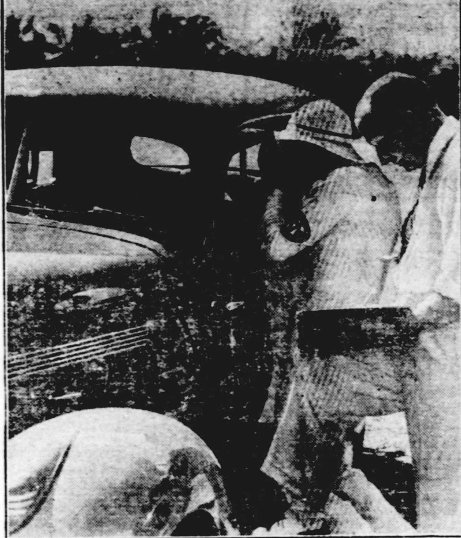
Stanley L. Reed, technical representative of the American Automobile Association contest board, takes a reading from the thermometer suspended inside after lengthy exposure of this General Motors car to the tropical Key West sun. He is being assisted by Kaye Don, noted British sportsman, who is recording the findings. Ability of the seamless steel roof of the Fisher "turret top" body to deflect the sun's rays accounts in part for the fact that the interior temperature of cars equipped with it are less affected by atmospheric conditions than others, the tests show.
