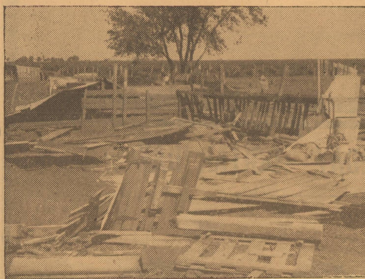
This is all that remained of the cow barn on the E. H. Meeks farm, in Oklahoma Lane community, when the twister struck there. It was a 15x40 frame structure and was located a few hundred feet south of the Meeks home.
