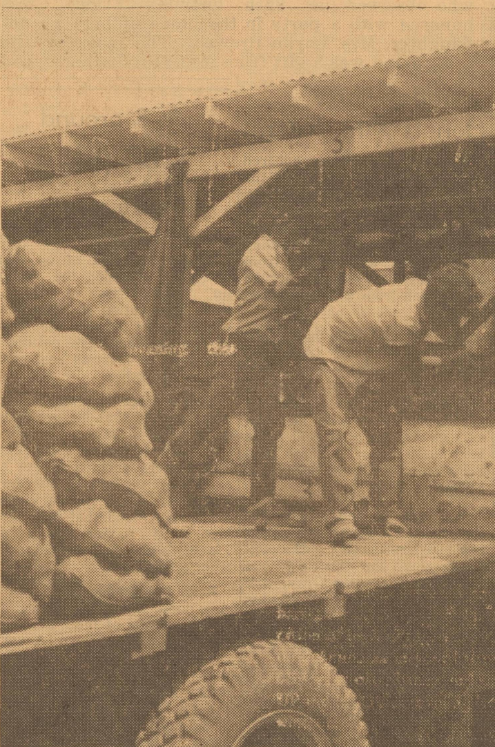
The first step in potato processing at Friona Growers & Shippers is to unload the spuds as they arrive from the field and dump them into these bins where they await their turn at the washing, grading, and packing operations.
