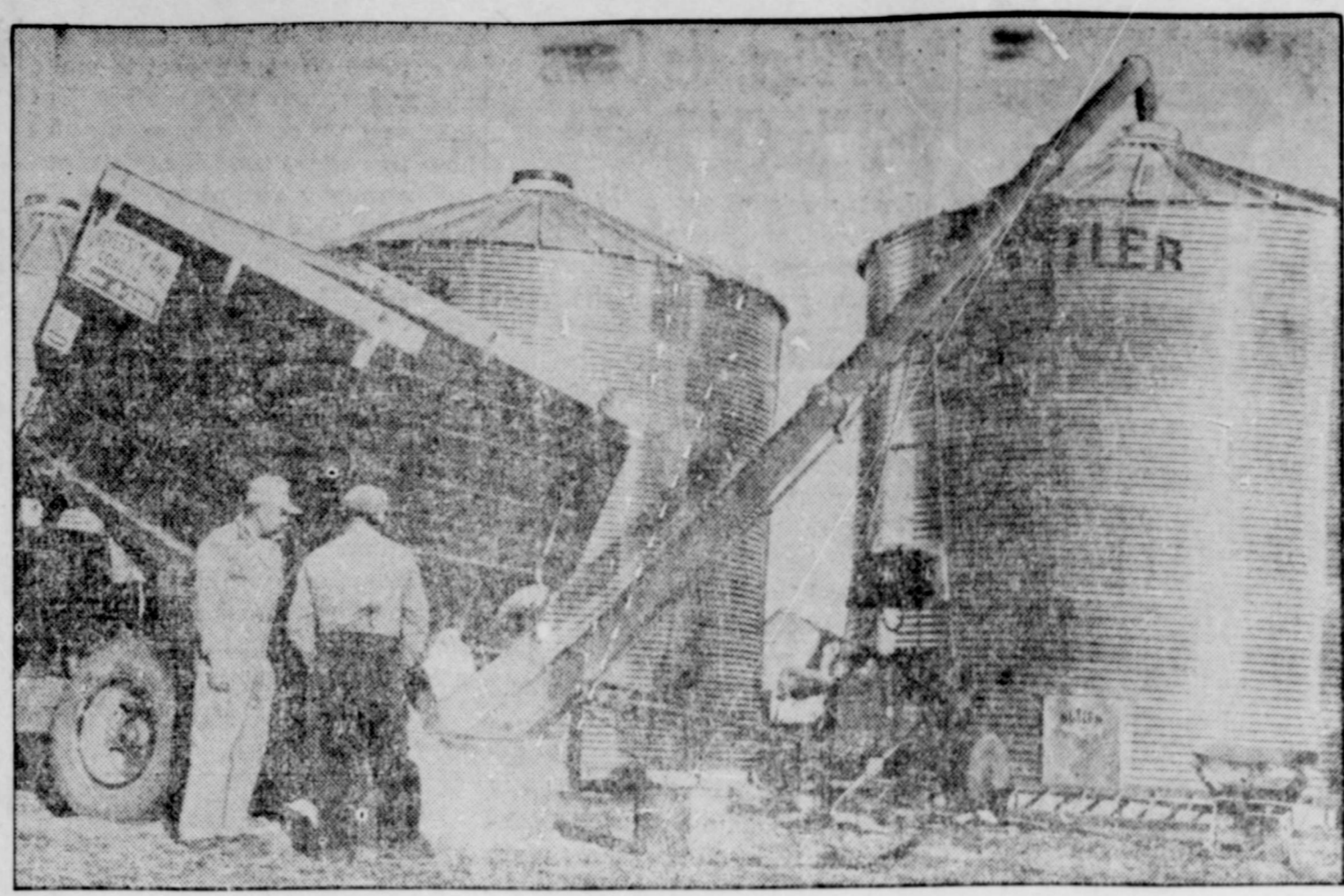
SAVING THE HARVEST —Farmers pour grain into one of the aluminum bins set up by the government at Enterprise, Iowa, to provide storage for the unexpectedly large 1949 grain harvest. About 26,000 bins were erected with an average capacity of 3250 bushels each to help meet the harvest emergency.
