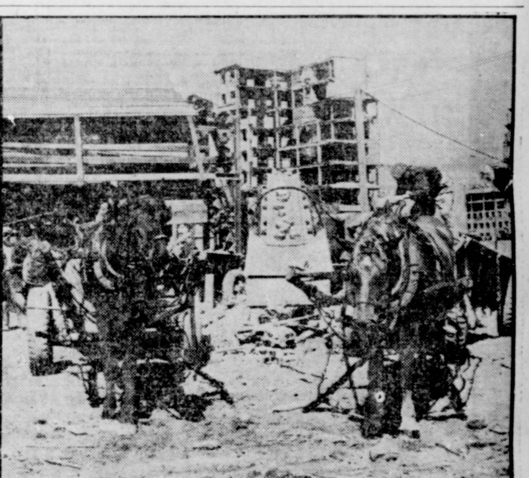
REBUILDING WARSAW—Rubble in war-torn Warsaw provides the bricks badly needed for the reconstruction of the city. Special mills, located near the devastated areas, are grinding and sorting the rubble for the concrete-making machines. The carts behind the horses are being loaded with rubble bound for the mill.
