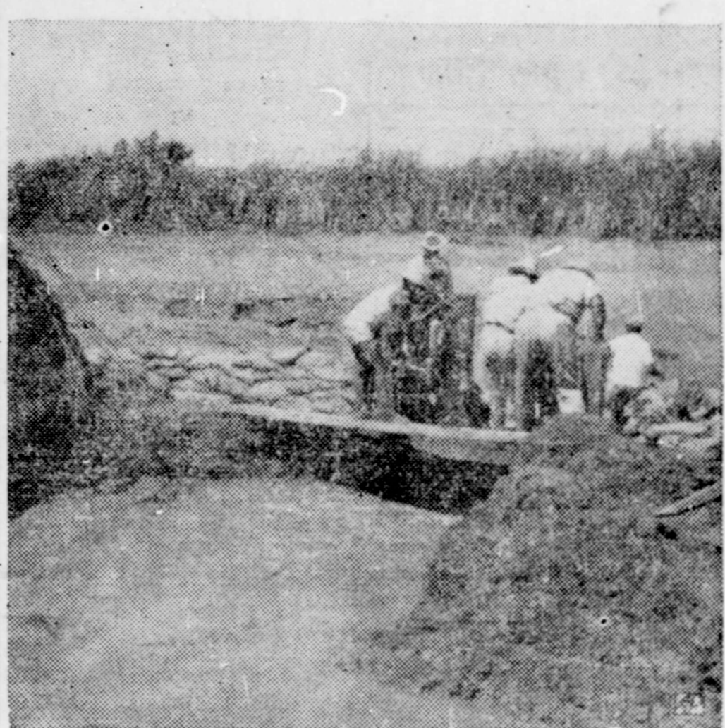
A break in the Mercedes irrigation district main canal left the south Texas city without water. Above, workmen rush to repair the break in the canal bank. Emergency water supplies were trucked to Mercedes. Fishermen had a holiday harvesting striped gar and catfish with pitchforks and machetes. (AP Photo).
