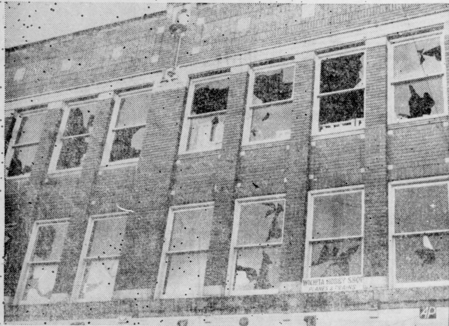
Properly damaged totaled several hundred thousand dollars in Wichita Falls as hailstones the size of hens' eggs fell in the business district. Few windows on the top two floors of this building escaped destruction. (AP Photo)
