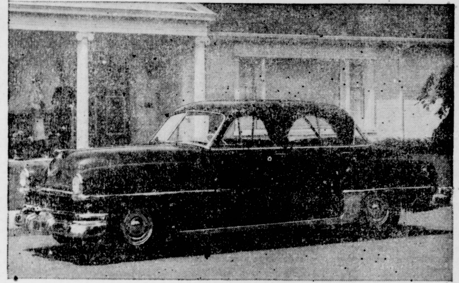
New in the 1951 Chrysler line is the Saratoga model powered by the 180-horsepower FirePower V-8 engine, which previously has been available only in the longer wheelbase New Yorker, Imperial and Crown Imperial models. With a wheelbase of 125½ inches, the Saratoga will be available in the six-passenger sedan pictured above, eight-passenger sedan, limousine, club coupe and the Town and Country wagon. Saratoga models will be available in a wide choice of standard colors and two tone color combinations.
