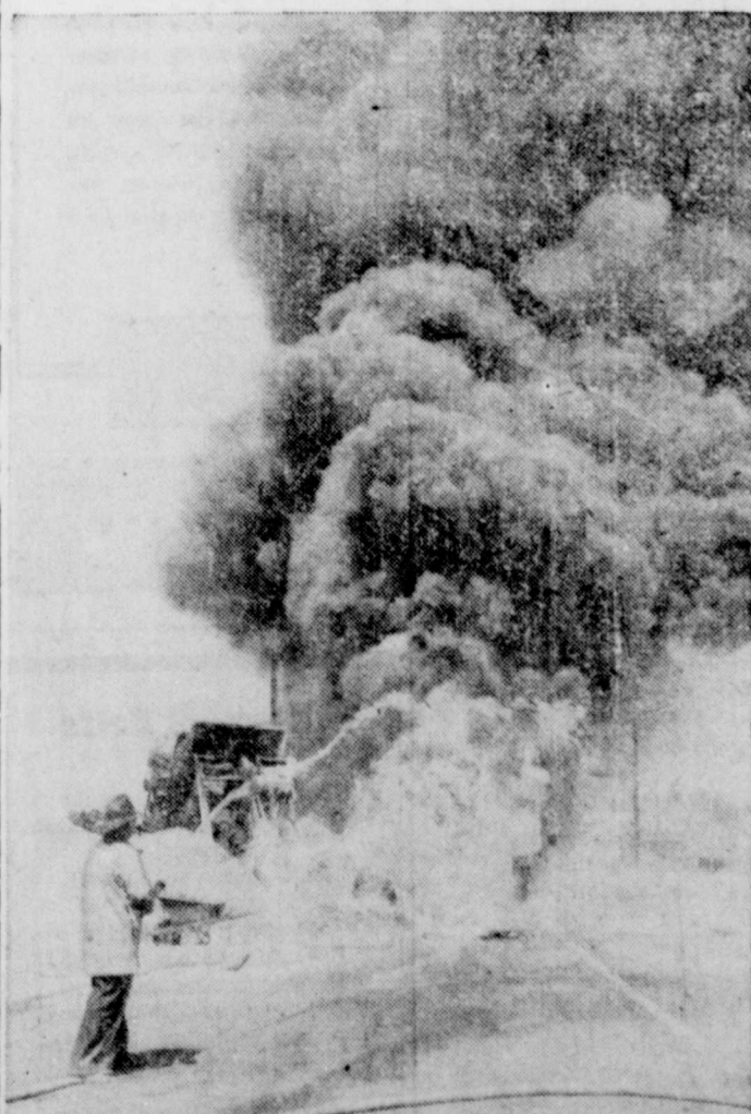
ALL UP IN SMOKE —A lone fireman sprays water on a burning trench-digging machine and gasoline pipe line in Los Angeles, Calif., after the machine accidentally cracked open the high test gasoline pipe line. The operator managed to climb to safety.
