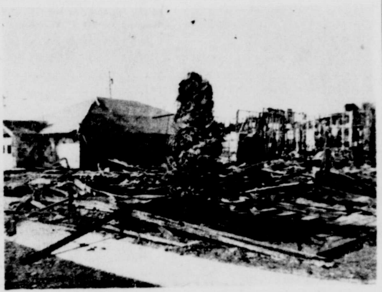
Pictured above is all that remained of the East Cisco Baptist Church after the devastating fire last week. Officers announced that a drive for funds to rebuild the structure would begin at services Sunday.
