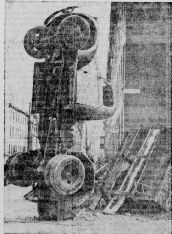
NICE ON A COLD DAY—The driver of this truck in Philadelphia, Pa., was supposed to be using the dump truck to deliver a load of coal. When he went around a corner, the weight of the coal called the turn, set the driver on his back, spilled out then and there and delivered the driver unhurt but riding high. And that settles the question of which end was running the truck.
