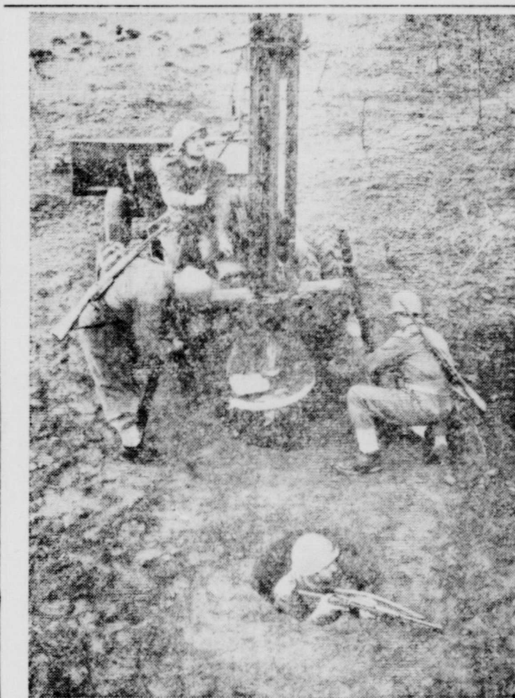
EXCAVATOR FROM HEAVEN—No longer will tired infantrymen have to dig foxholes when they get into action. Italian Army engineers, shown in Rome, have designed a machine capable of digging an eight-foot hole in less than two minutes. Above, a soldier holds guard position in a newly-dug foxhole while the digging machine excavates another one nearby.
