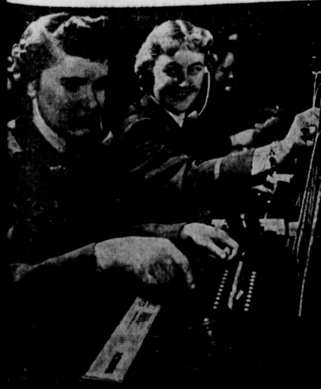
WOMEN OF THREE NATIONS work and live together at SHAPE. In the photo above, Corporal Irene Croft, U.S. Army WAC, Idaho, left, and Sergeant Janine Yovanovitch of France at the central switchboard. Dutch WAC's work with them.
