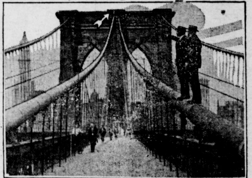
That largest suspension span on the famous old structure, the Brooklyn Bridge at New York, has slipped under the constant hammering of traffic and authorities have closed it to all except pedestrians. Arrow points to slipping cable.
