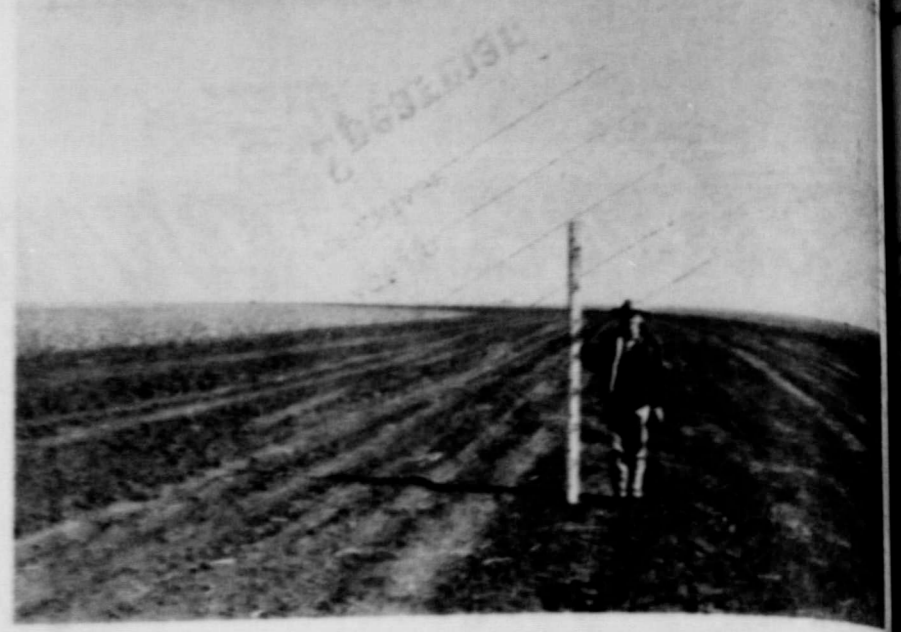
A DIVERSION TERRACE HAS JUST BEEN CONSTRUCTED ON THE INEZ BENNETT FARM. Technical assistance and cost share is available on such conservation practices as irrigation pipeline, land leveling, livestock water wells, waterways, ponds, terraces and grass planting through the CFCP and the ACP Programs. The Soil Conservation District provides planning, layout, and construction checks on such conservation work.
