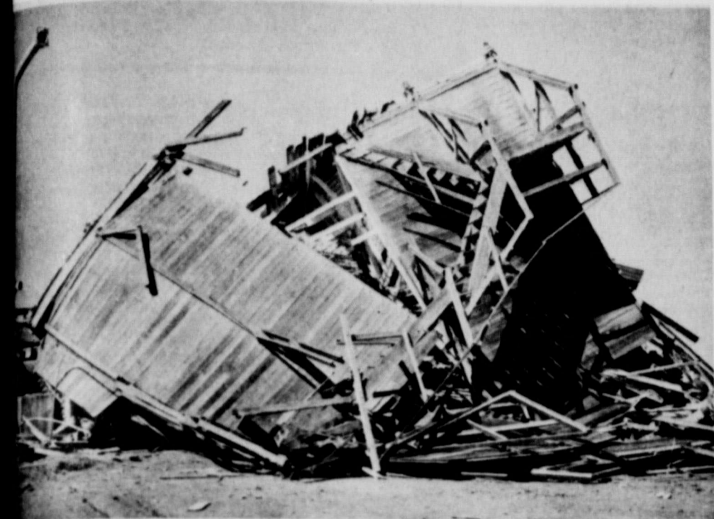
Northern Natural's Cooling Tower
