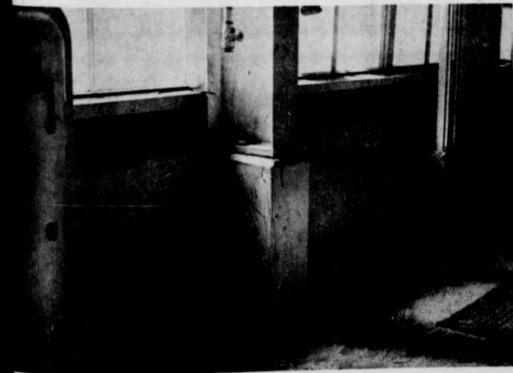
Steel and Cement give way to tornadic winds
