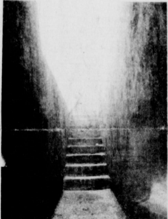
THIS SHOT OF the cattle dipping vat for scabies control is taken from down inside the pit. Cattle will swim through the liquid and out this end. Dee Allen is building this public facility to state specifications with a declaration that the vat may be used for all county cattle at a reasonable price. The state has directed that such a vat be located in every county to help control the current scabies outbreak.
