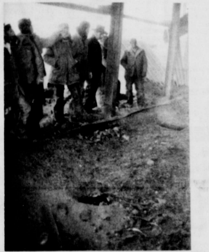
THIS IS ALL that was left after the explosion at the feed mill load-out area. This was once truck scales, set in a 10x50 foot concrete slab. Gas trapped under this scale is thought to have caused the explosion.
