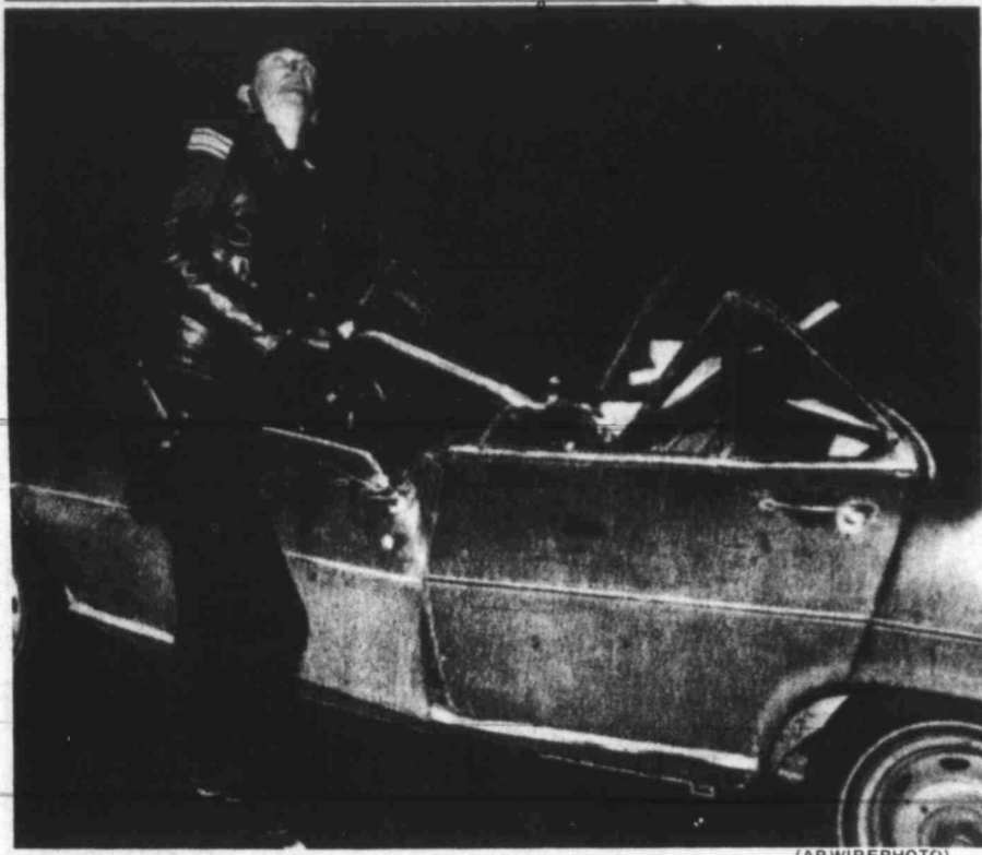
THE MARBLE'S MARK — Slab of marble which fell from facade high up on 74-story Water Tower Place in Chicago did this damage to car of Dr. Martin Brandfonbrener, 48, of Winnetka, a Chicago suburb. Brandfonbrener got two broken ribs. The slab weighed 250 pounds, and fell behind his driving position.
