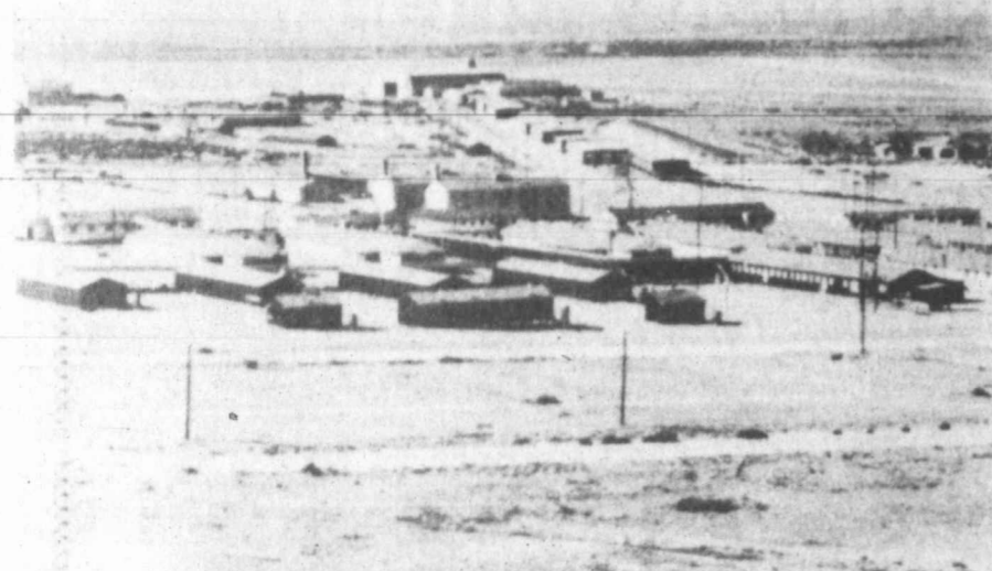
NEW CAMPUS — Howard Junior College hopes to be moved into the Bombardier School buildings by September and begin classes for the newest junior college in Texas.
