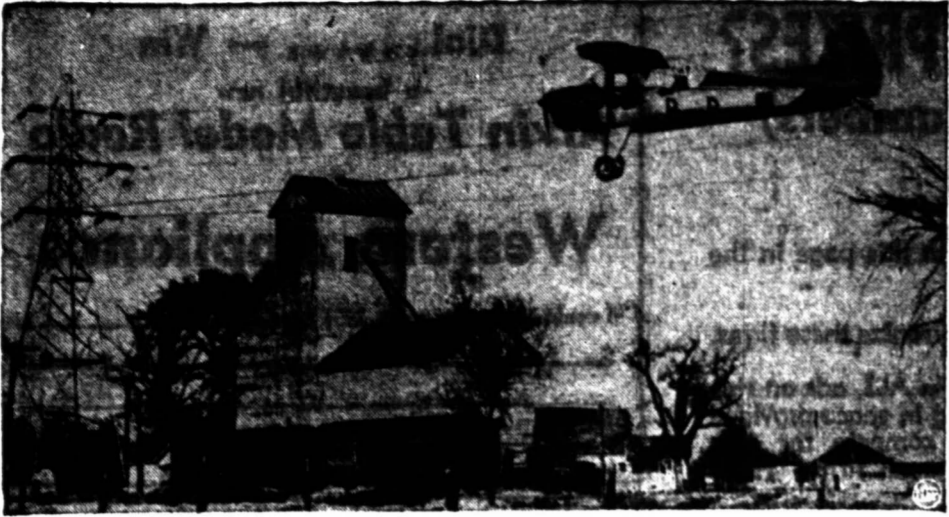
FLYING LINEMAN —Modern methods are speeding up inspection of electric power lines. The Illinois Power Company now uses planes of a "Power Patrol" to skim alongside its lines, looking for trouble. The composite photo shows how it's done.
