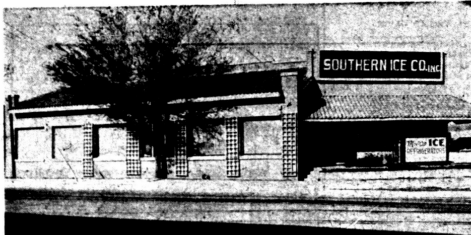
FOR WINTER DESSERTS —Manufactured ice is a "must" for winter desserts and other iced delicacies, and the Southern Ice Company, 310 South Main Street, is equipped for the most rapid and convenient servicing of your ice needs. The dock is especially constructed for the convenience of customers.
