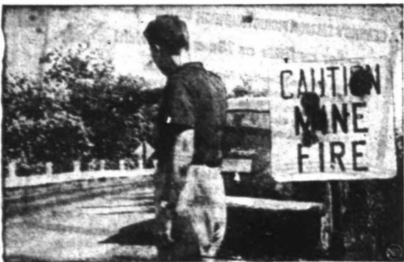
Roadside warning is necessary on New Stratsville highway, recently patched after cave-in caused by underground fire.
