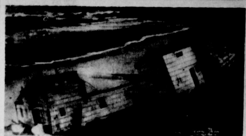
LEAVING LANDS END... Landslides send Sea Gull cottages sliding to beach at Lands End, Ore., caused by heavy rainfall. Heavy rains and floods have been inflicting heavy damage in northwestern Oregon.
