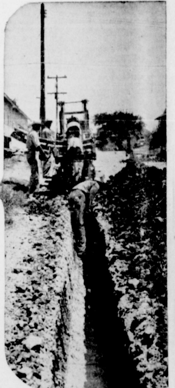
Ditching machine is major unit of highly mechanized teams who build new distribution lines in towns and cities on Lone Star Gas System.
