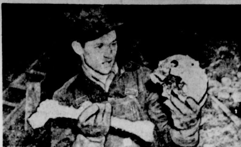
'WHODUNNIT'... Washington, D.C., construction worker examines skull and bone of a man found by excavators sunk in lime. Police said skull had been "bashed in."
