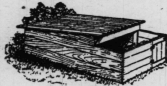
The Hog House in Position.
