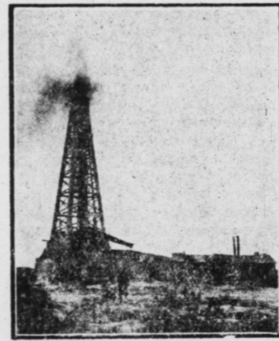
S. E. 1/4 SECTION 8, BLOCK 59, SCHOOL SURVEY, REEVES COUNTY. STANDING 600 FEET IN OIL AFTER SHOOTING WITH 250 QUARTS OF NITROGLYCERINE AT 1950 FEET.
