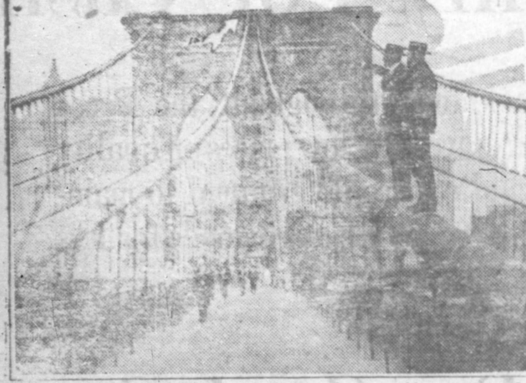
The largest suspension span on the famous old structure, the Brooklyn Bridge at New York, has slipped under the constant hammering of traffic and authorities have closed it to all except pedestrians. Arrow points to slipping cable.
