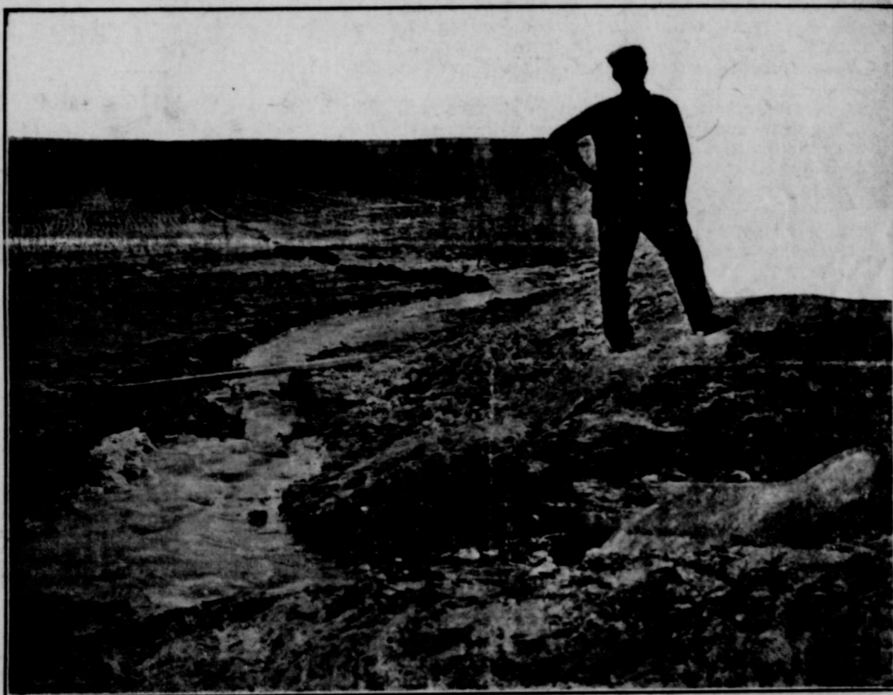
This is a sample of our waterworks, a Scheme
