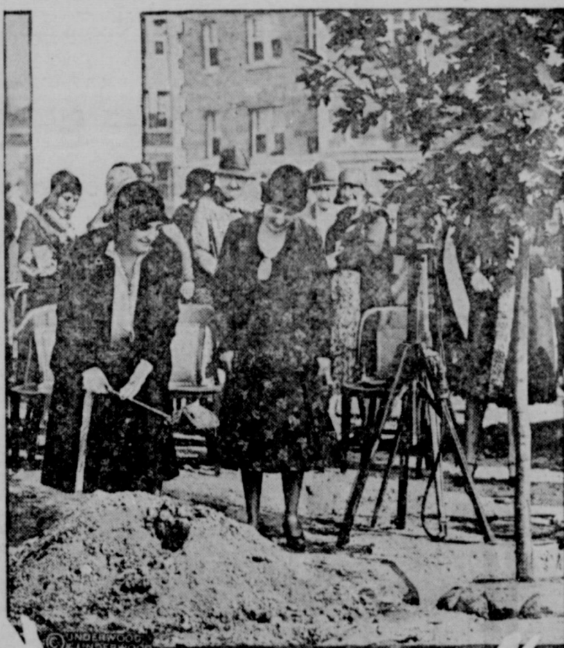
Mrs. Herbert Hoover placing the first shovel of earth about the roots of a young maple tree on the newly constructed R. B. Murch school in Washington.
