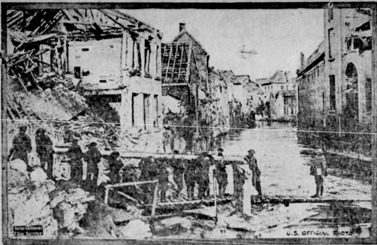
Members of C company, Three Hundred and Sixteenth engineers, placing the abutment for a bridge over the canal at Audenarde, Belgium.
