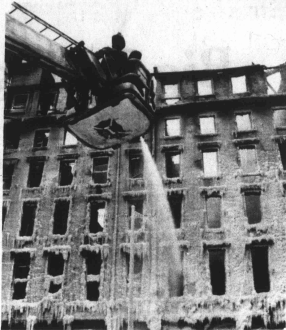
FAÇADE OF FROST — New York City firemen play stream of water on smoldering building, already ice-covered in the Greenwich Village section of New York City Sunday. Fire fighters had been spraying the building since it first erupted in flame Wednesday night. Frigid temperatures coated the fire-blackened facade with white frost during the wet-down period.
