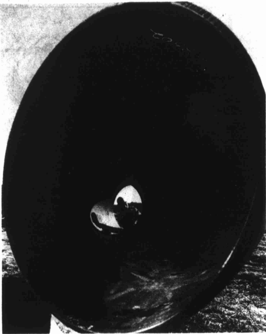
CLOSE QUARTERS — Andrew Balthazar, a welding inspector at Natchitoches, La., for Tenneco's Tennessee Gas Pipeline Company, works in close quarters as he checks the welds in a piece of pipe being readied for installation. In fact, it takes a bit of tunnel vision to see him at all.
