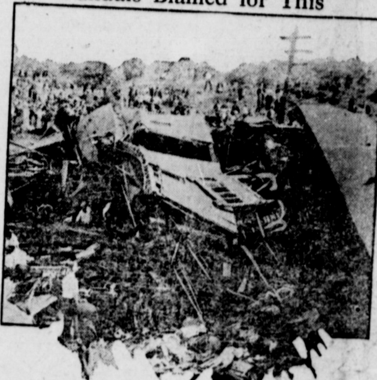
Detectives say this wreck of a New York-Chicago express on the Michigan Central at Gary, Ind., was caused by vandals who pulled up spikes. Two were killed and two seriously injured.
