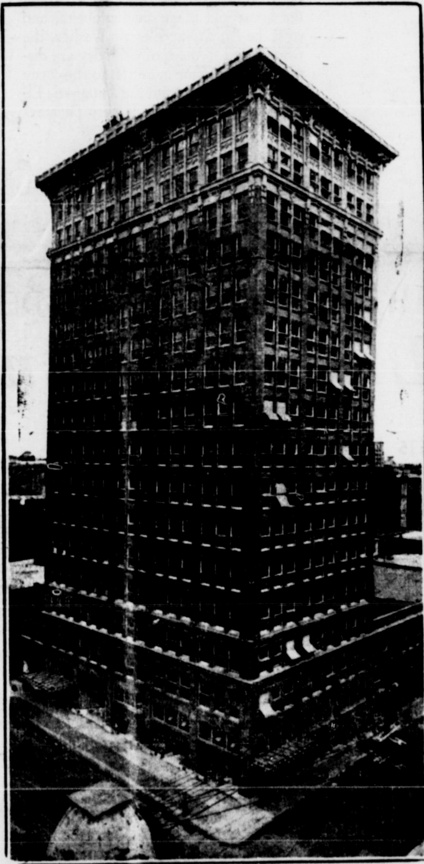
SOUTHWESTERN LIFE BUILDING Dallas, Texas
