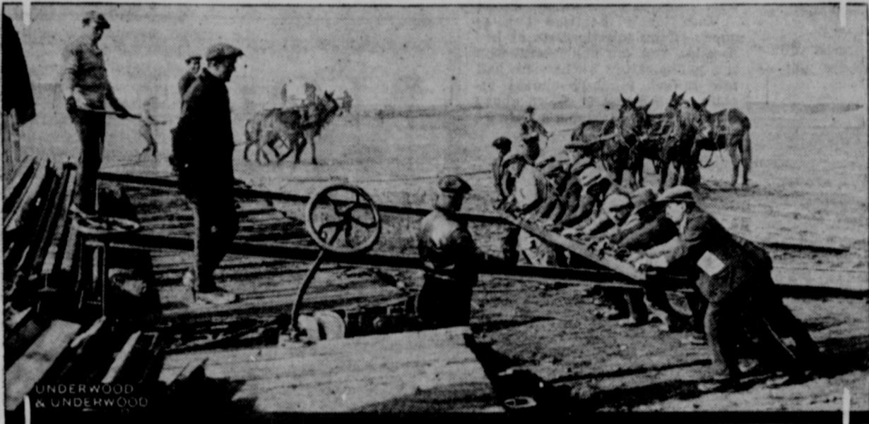
What was said to be the shortest railroad in the world, running for one and one-half miles between the docks and warehouses on Governors Island, has been condemned by the United States army and torn up. Built during the war to transport stores and machinery on the island, the railway, with the official name Governors Island railroad, gradually decreased in usefulness.
