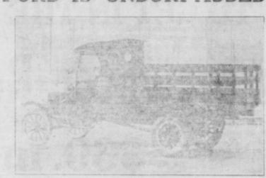
is is the new stake body produced by the Ford Motor Company or its one ton truck. It is designed to meet a wide variety of trucking requirements both in the commercial and agricultural indi. Exception the floor and rack boards, the body is all steel
